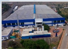
TATA TOYO RADIATOR LIMITED
